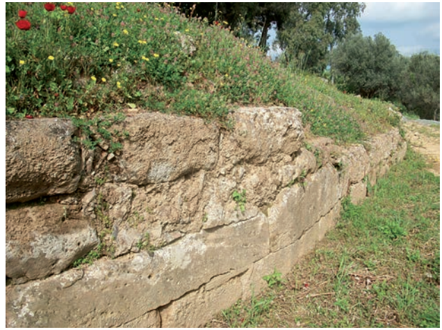
Fig. 5. View of the retaining wall of the terrace (photo: G. Alevras).
