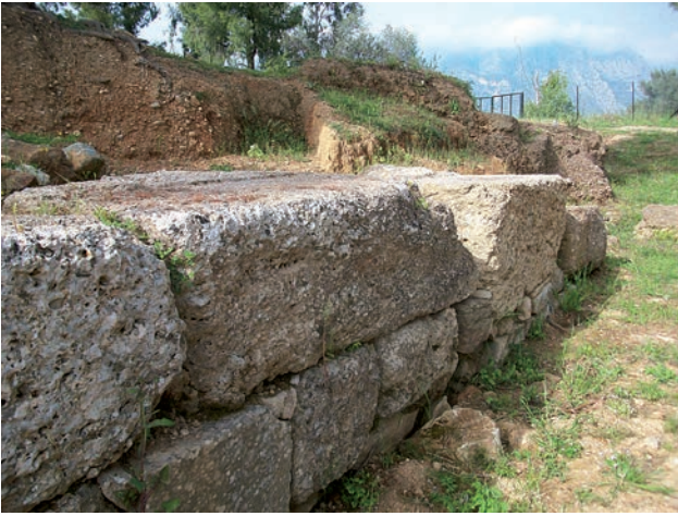
Fig. 4. View of the retaining wall of the terrace (photo: G. Alevras).
