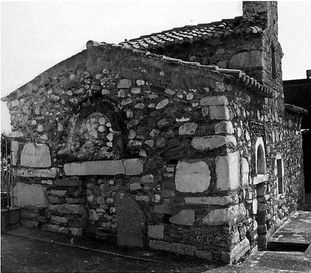
Fig. 3. Architectural members of the throne and altar that were walled into the church of Profitis Ilias (photo: Stavros Vlizon).
